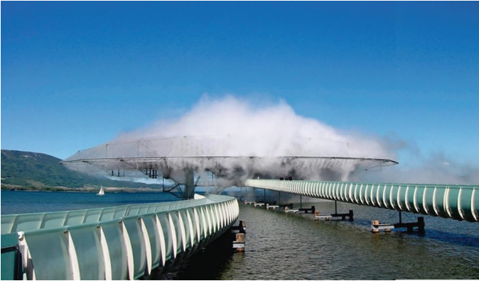
Figure 7. Blur Building, Yverdon-les-Bains, Switzerland. Designed by Diller Scofidio + Renfro for the Swiss Expo 2002, the Blur Building uses a system of high-pressure nozzles to create an artificial cloud suspended over Lake Neuchâtel. By obscuring vision and dissolving architectural form into atmosphere, the building compels visitors to rely on sound, touch, and bodily perception. This sensory recalibration challenges the primacy of vision in architecture and redefines the relationship between humans, space, and environment. The figure is reproduced from Reference 29.
