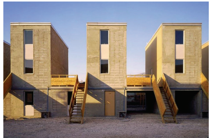
Figure 4. Quinta Monroy Housing Project, Iquique, Chile. Designed by Alejandro Aravena and ELEMENTAL in 2003, Quinta Monroy provided low-income families with affordable starter homes that deliberately left half of the structure unfinished. This approach empowered residents to expand and customize their houses over time, making them co-creators of their living environment and fostering a sense of ownership and community. The figure is reproduced from Reference 20.
