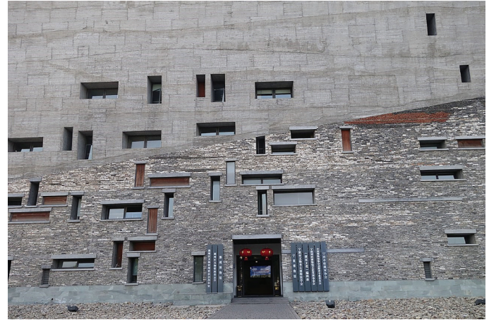
Figure 8. Ningbo Museum, Ningbo, China. Designed by Wang Shu and completed in 2008, the Ningbo Museum incorporates old bricks and tiles salvaged from demolished local villages. This reuse of vernacular materials embeds layers of history and memory into the building, encouraging visitors to connect emotionally with the past. Beyond aesthetics, the design exemplifies respect for cultural continuity and collective identity. The figure is reproduced from Reference 30.
